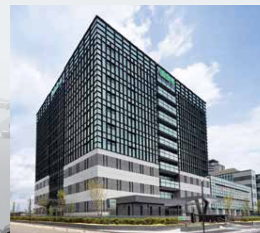
NIDEC ADVANCE TECHNOLOGY CORPORATION (Headquarters/Factory)
